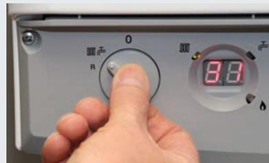
Turn on selector switch (display will show boiler temperature).
