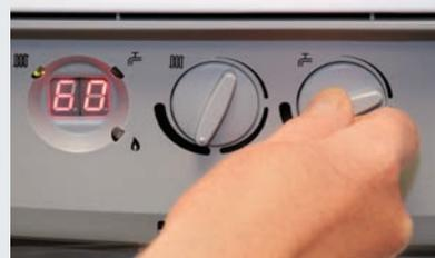
Set the clock and adjust the tappets to select the periods you require the heating to be on for. Timer options are: Off, Timed or Constant.
